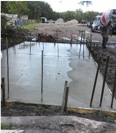
Dumpster Pad Poured
