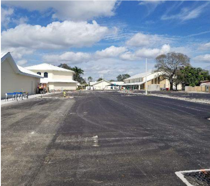
Parking Lot Paved
