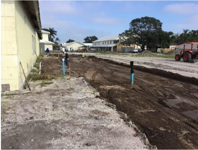
Grading in Progress
