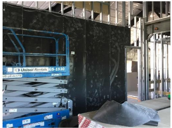
Sound Membrane Installed
