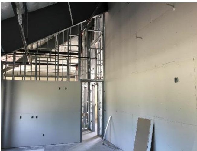
Select Drywall In Progress
