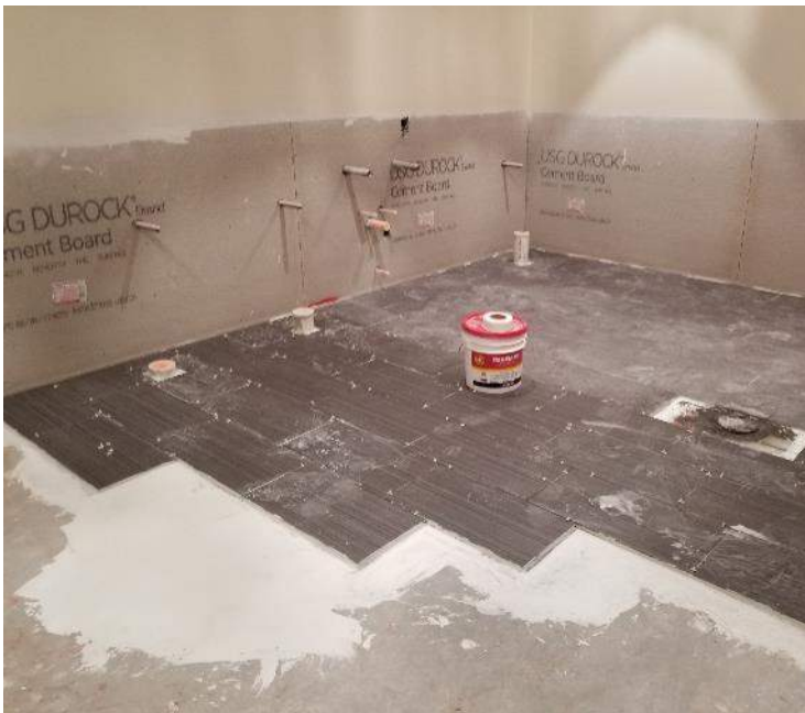
Floor Tile in Progress
