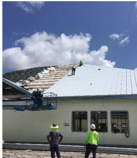
West Roof in Progress
