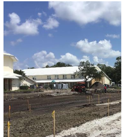
Parking Lot Grading
