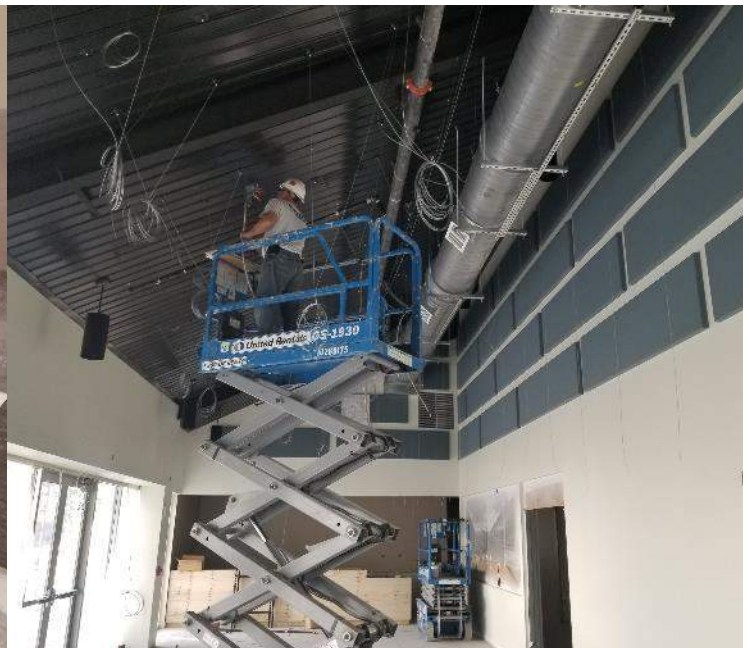
Entry Room Progress
