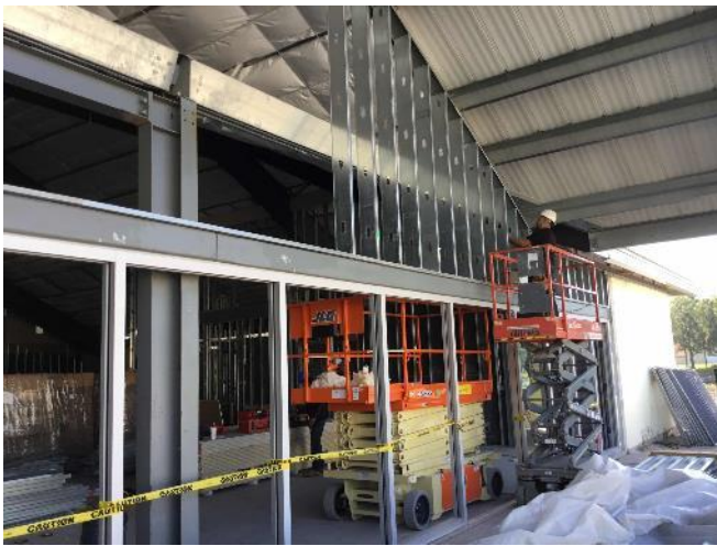
Exterior Storefront and Framing
