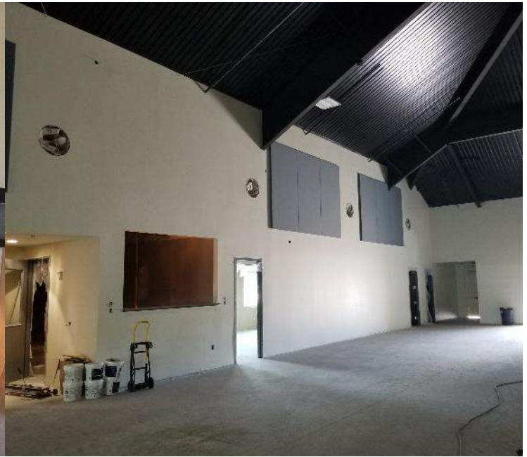
Sound Panels in Progress
