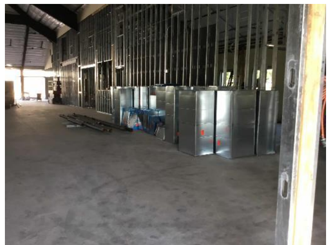
Ductwork in Progress
