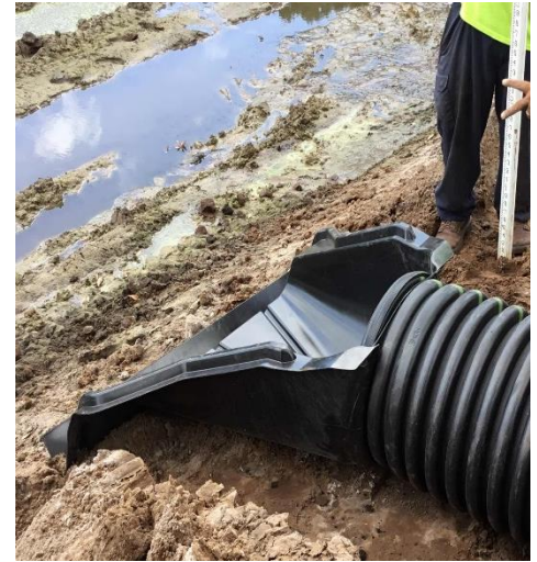
Flared-end storm pipe installed
