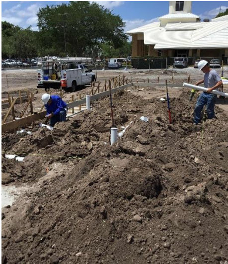
Plumbing Rough In
